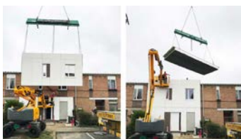
Energiesprong, Wattrelos, Red cat architecture, 2022
